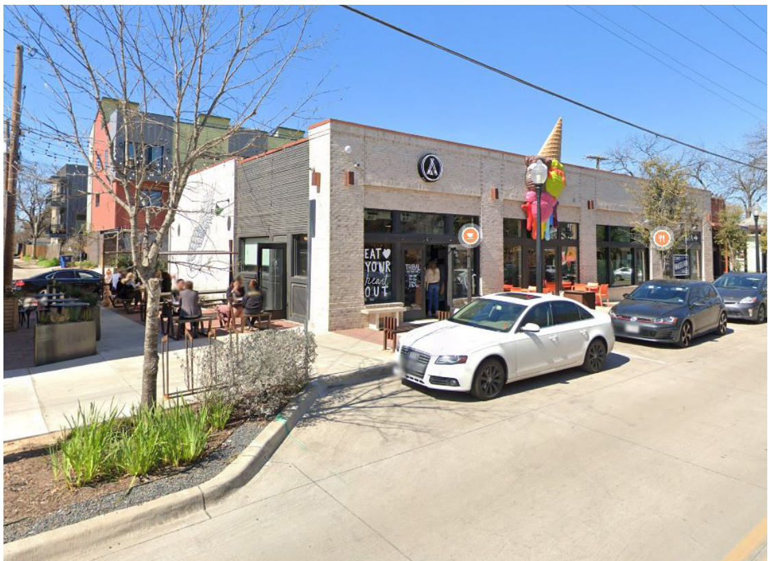
Single-story walkable retail format building in Bishop Arts by Exxir Capital Retail assessed at $218/sf Floor Area (2020)
