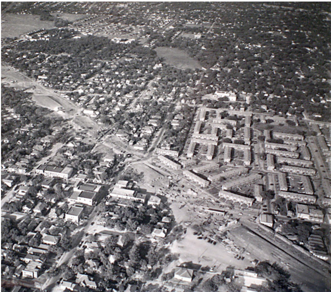
The clearing of land through the State-Thomas neighborhood for the construction of US75
