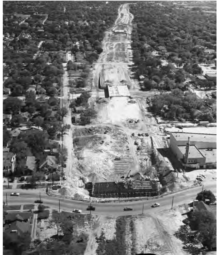
The Central Expressway under construction.
