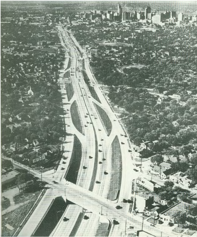
The Central Expressway shortly after opening.
